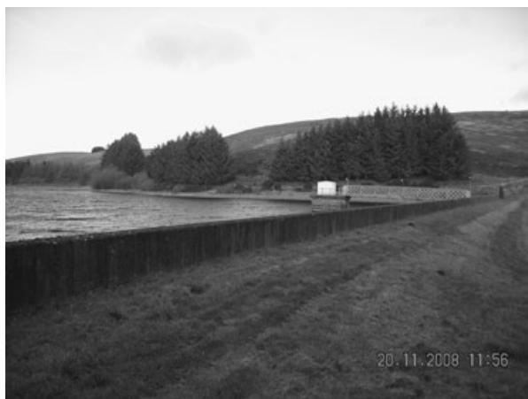
Fig. 4. Glenfarg Reservoir (near to Rossie Ochill, County of Perth and Kinross), an example of a Traditional Flood Retention Basin (type 2) that is, however, currently used only for drinking water supply purposes (picture taken by Qinli Yang on 20 November 2008).
